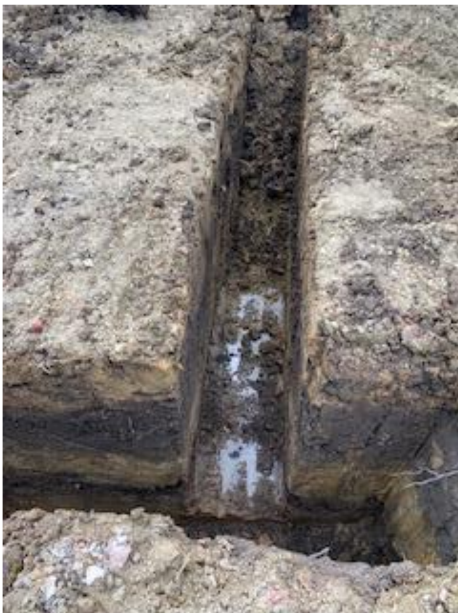
Plate 4. Typical section across site with deposited subsoil (Clay) overlaying topsoil (looking SSW)
