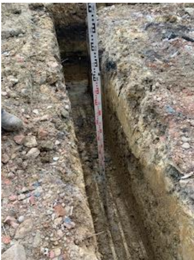
Plate 2. Depth of foundation cut- 1.3m
